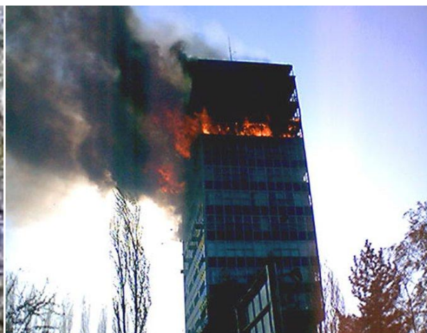
Figure 8b: The rapid spread of fire to other floors
