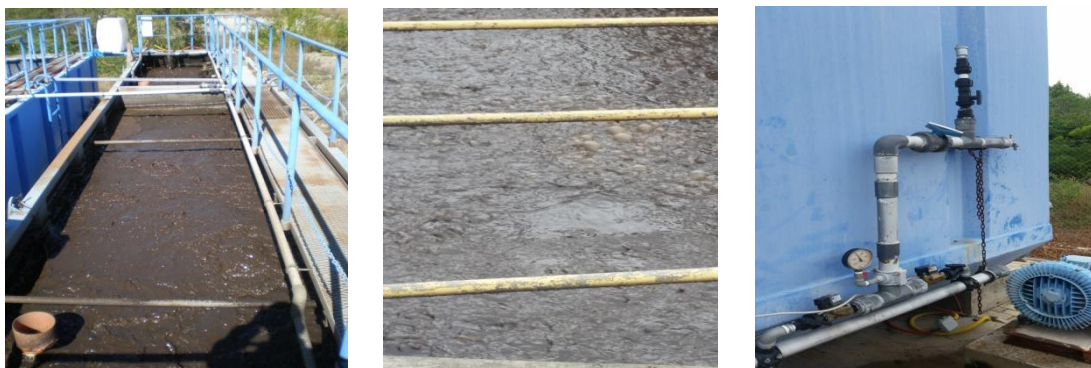
Figure 3. Part of the biological reactor sample points and effluent sample taken point
